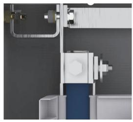
5 : Proceed to terminate the phase cores. An example configuration is shown below. Due to the lay of the cores on any one installation, this exact situation may not be achievable. The 'U' shaped lateral extension effectively enables a flexible 'third' position and is provided for this purpose. It is best used in either the Brown or Black phase position.
