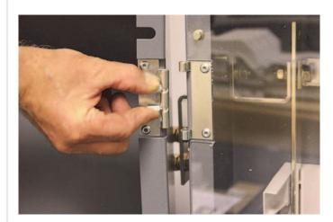
3 : Carefully remove all the clear covers from inside the SMDB by pulling on the black plastic fasteners. Take out the 'J' type fuse handles and loose stowed components including cable connectors and assorted fixings. For removal of the fuse handles, see section "6.6 Fuse Handle".
