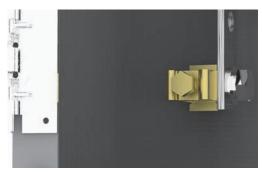
2: The fourth (neutral) core must be straightened dressed and terminated prior to the phase cores as it runs under them in the neutral channel situated on the outboard edge of the cabinet. Attach the short stand-off length of copper using the M10 fixings supplied using the M10 hole. The stand-off must be placed on the inboard edge of the main neutral busbar as shown in the vertical position. **This connection must be tightened to 45Nm.**
