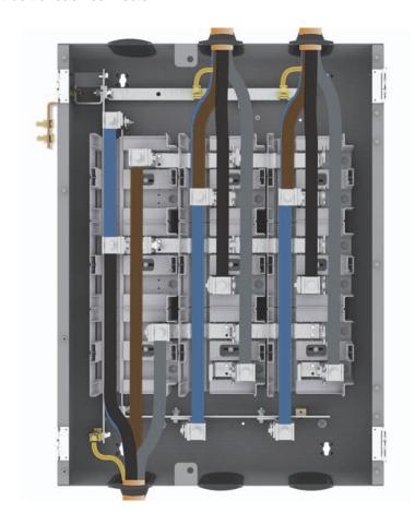
8: When all the cables have been terminated and the appropriate cable identifications have been added, proceed to conduct final polarity and continuity tests. With these satisfactorily completed, all the covers can be refitted.
