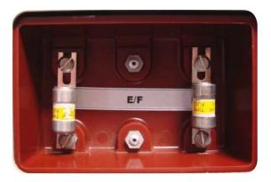
Fuse dimensions: Length 57mm x Diameter 13mm
